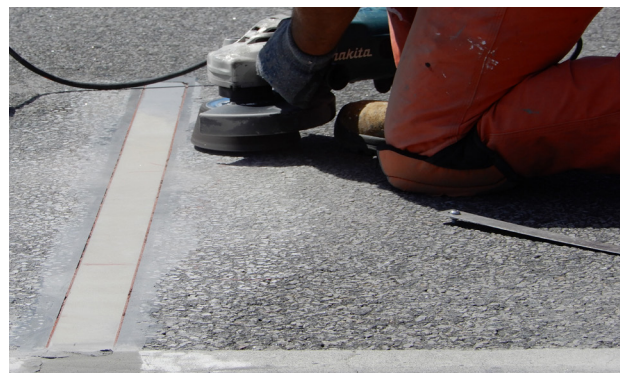
Sensors are installed in the pavement and ground flush with the roadway surface.
